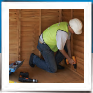
Insured installation crews
